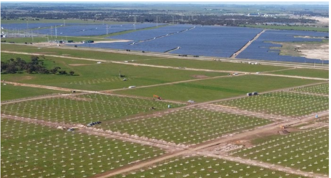
Tailem Bend 2 Project currently under construction in South Australia
