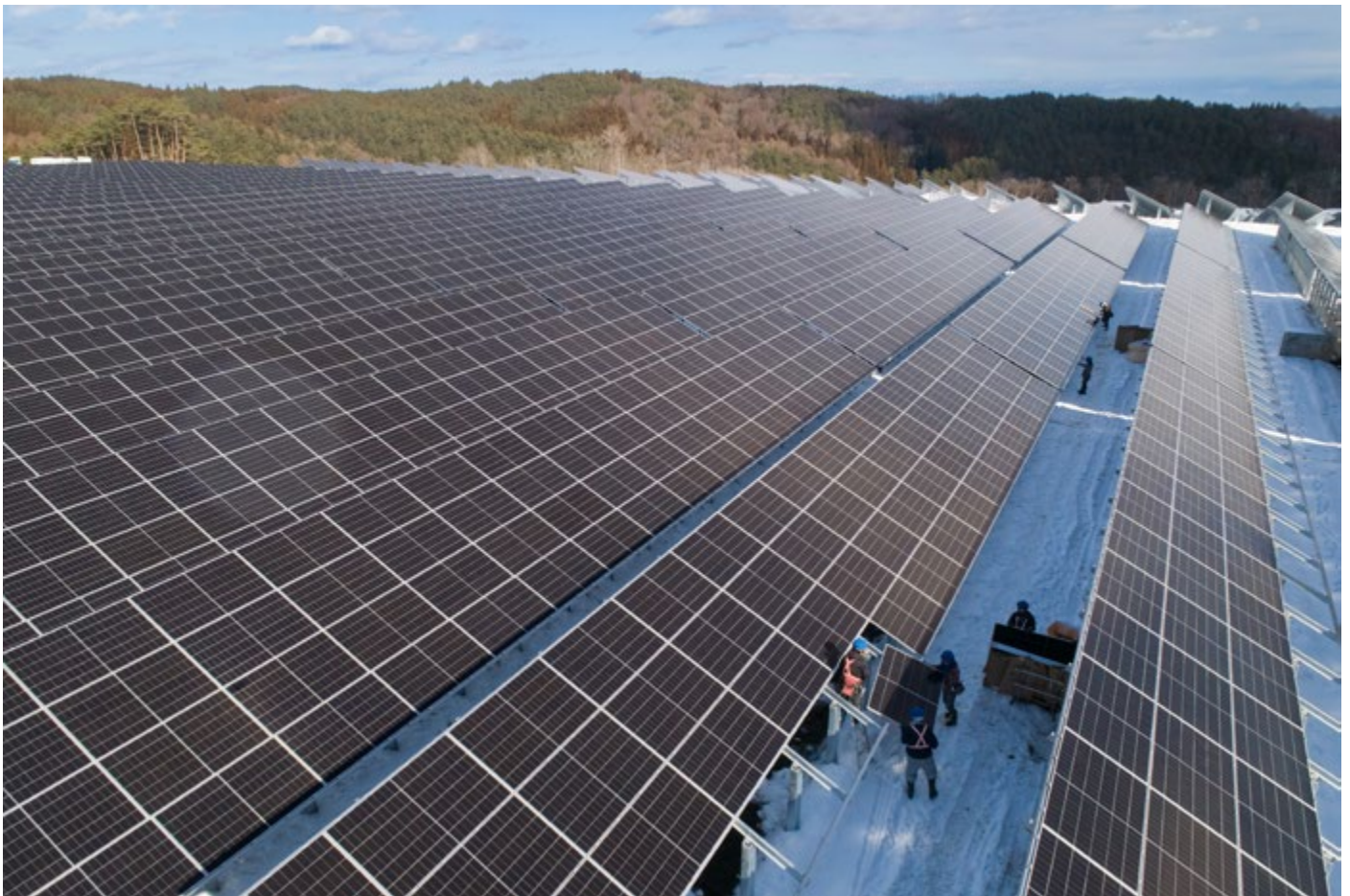
Installation of solar PV panels in Japan
